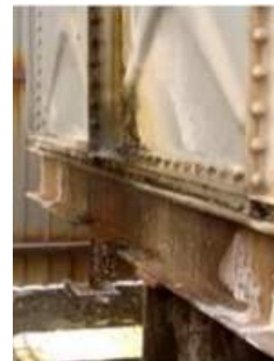
Images of corrosion previously documented
